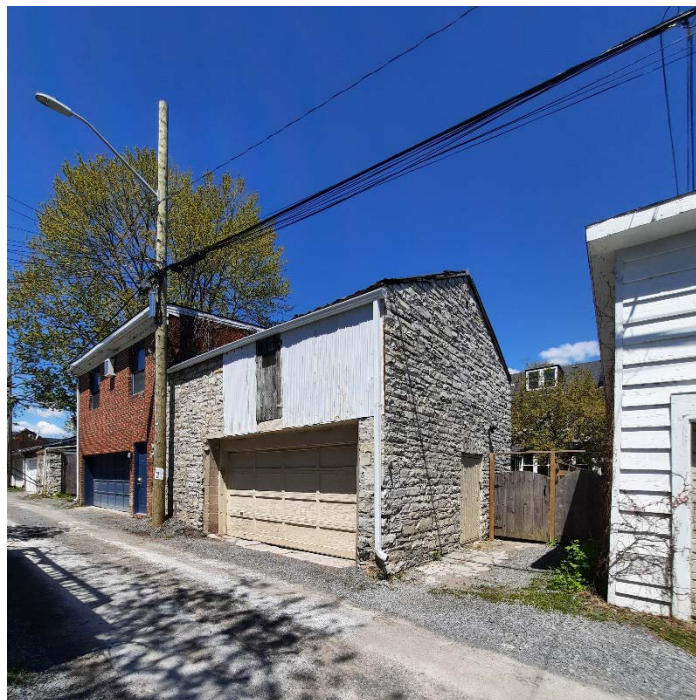
Outbuilding at 274 Johnson Street
