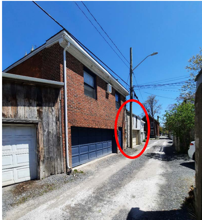
View looking east along laneway with 274 Johnson St. outbuilding in background
