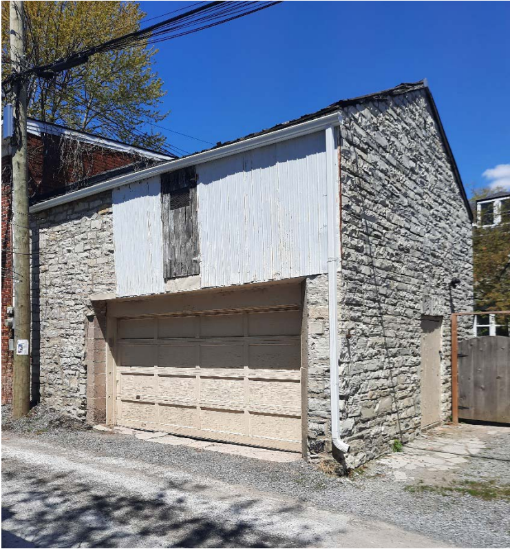
South elevation of outbuilding at 274 Johnson Street
