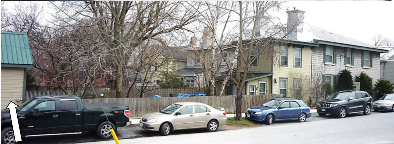
1, 1A, AND STUDIO ON Church Street – Porstmouth Village
