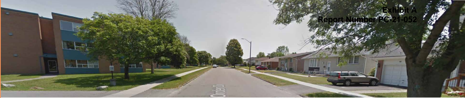
Figure 2-17: Calvin Park streetview showing student housing opposite residences (Google)
