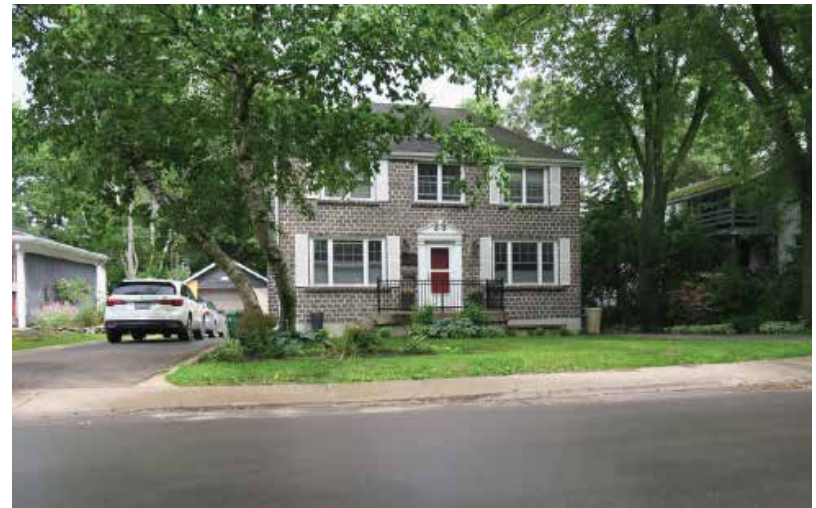
Figure 2-10: Typical single detached house in Group 2
