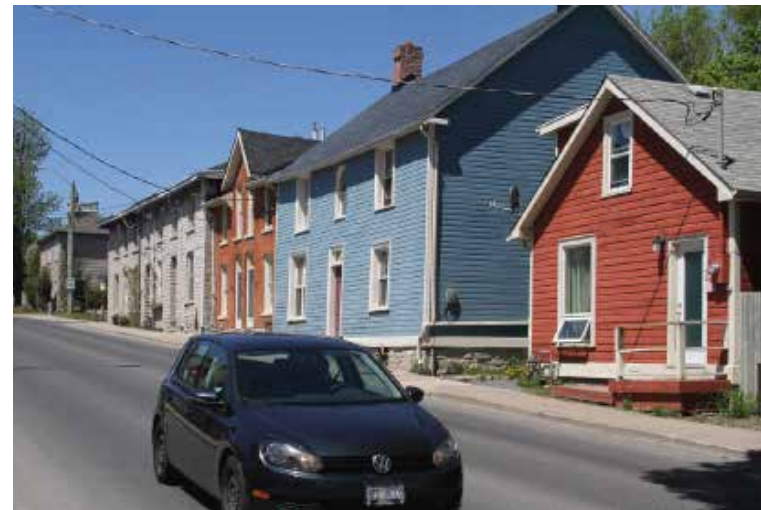
Figure 2-15: Street-oriented heritage buildings at the sidewalk in Portsmouth
