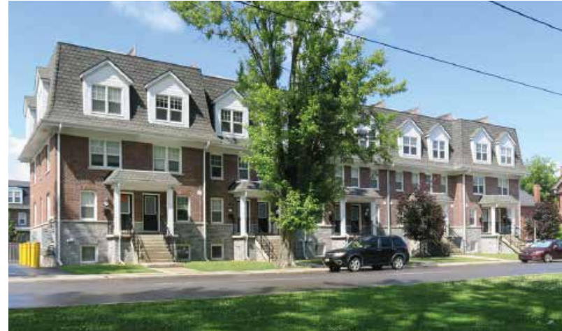
Figure 2-17: Newer development project with a rhythm of front doors, porches and roof dormers in Group 4
