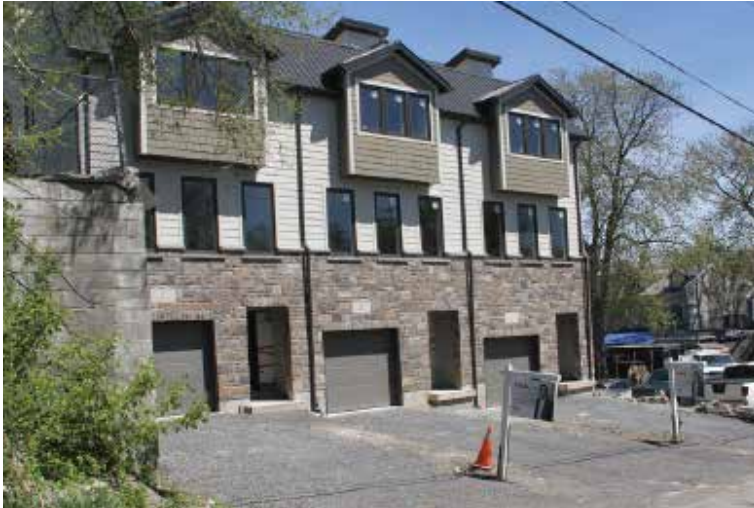
Figure 2-12: Newer development with front yard parking and garages in Group 3
