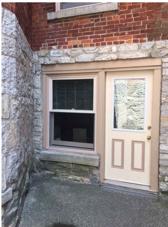
Figure 3: Existing Window and Back Door at 250-1 King St. E
