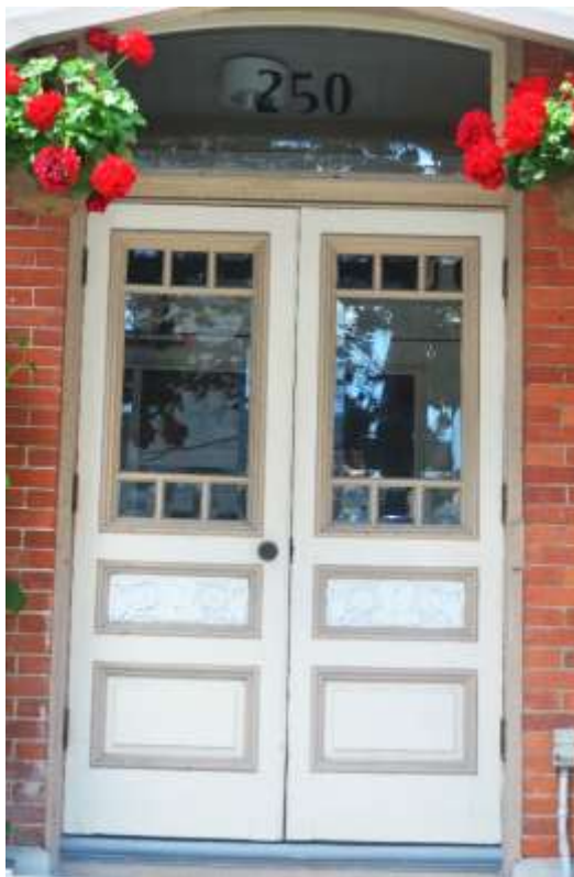
Photo A-6: 250 King St. E., Front door, Transom and Trim. 252 King St. E. is the same.
