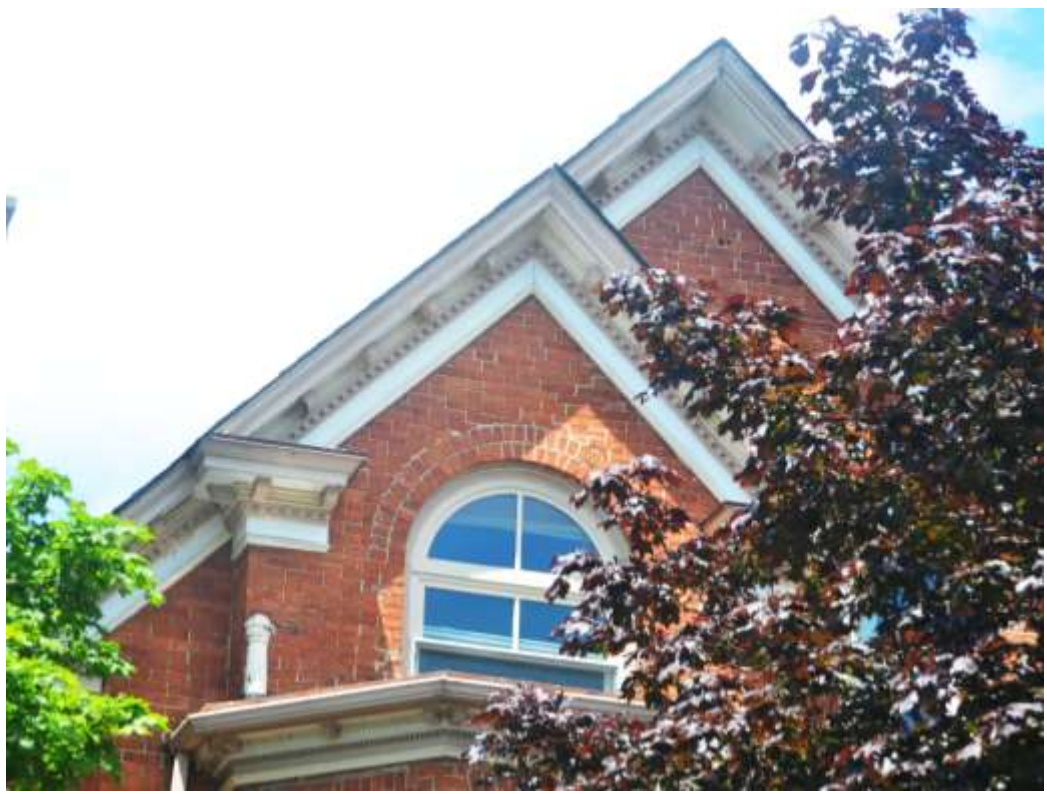
Photo A-8: 244-2 King St. E., Soffit, Fascia
