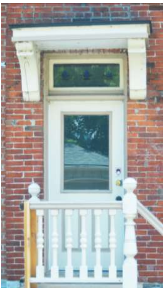
Photo A-19: 3-250 King St. E. Back Door, Transom and Trim, and Roof over Stoop. Same at 2-250 King. St. E and 3-41 William St.
