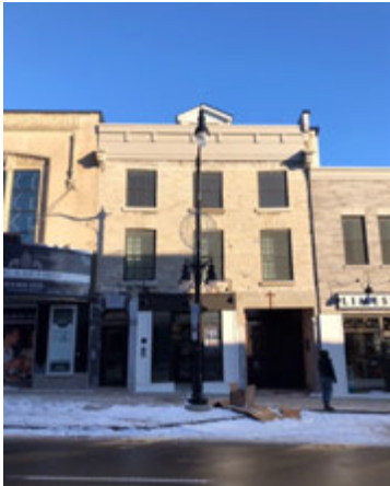
Figure 10: 219 Princess Street, Kingston. Adjacent listed property of cultural heritage value.
