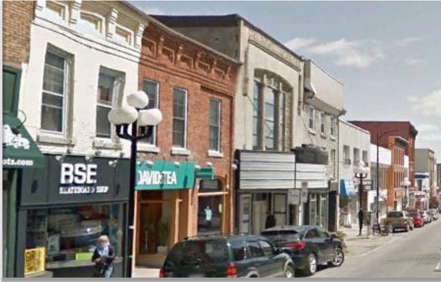
Image 7: Google Earth Street View Image c2011. Note altered roof and compare with Image 14 and 15. A second addition was added to the lobby c. 1967-73. Credit: Google Earth
