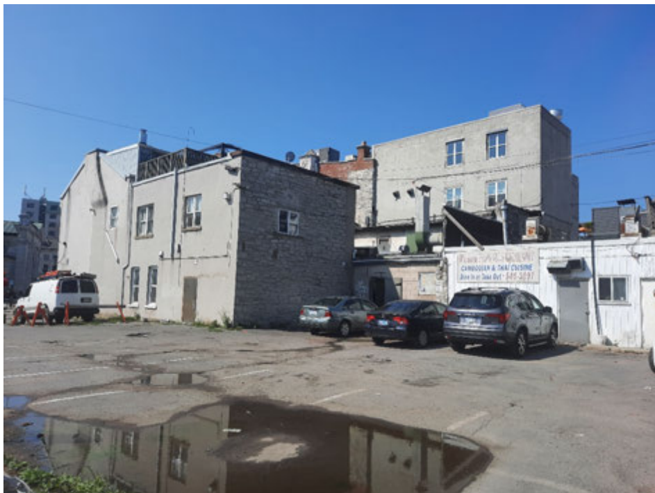
Rear of 35 Brock Street (Looking Southwest)
