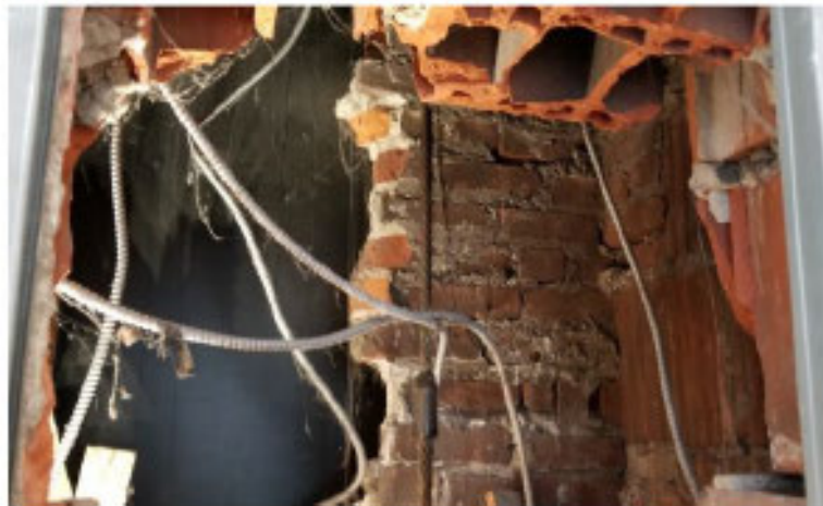
Photograph 3: Brick and block backing walls
