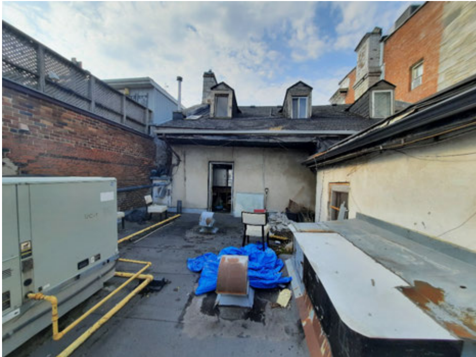
North Elevation at Second Floor
