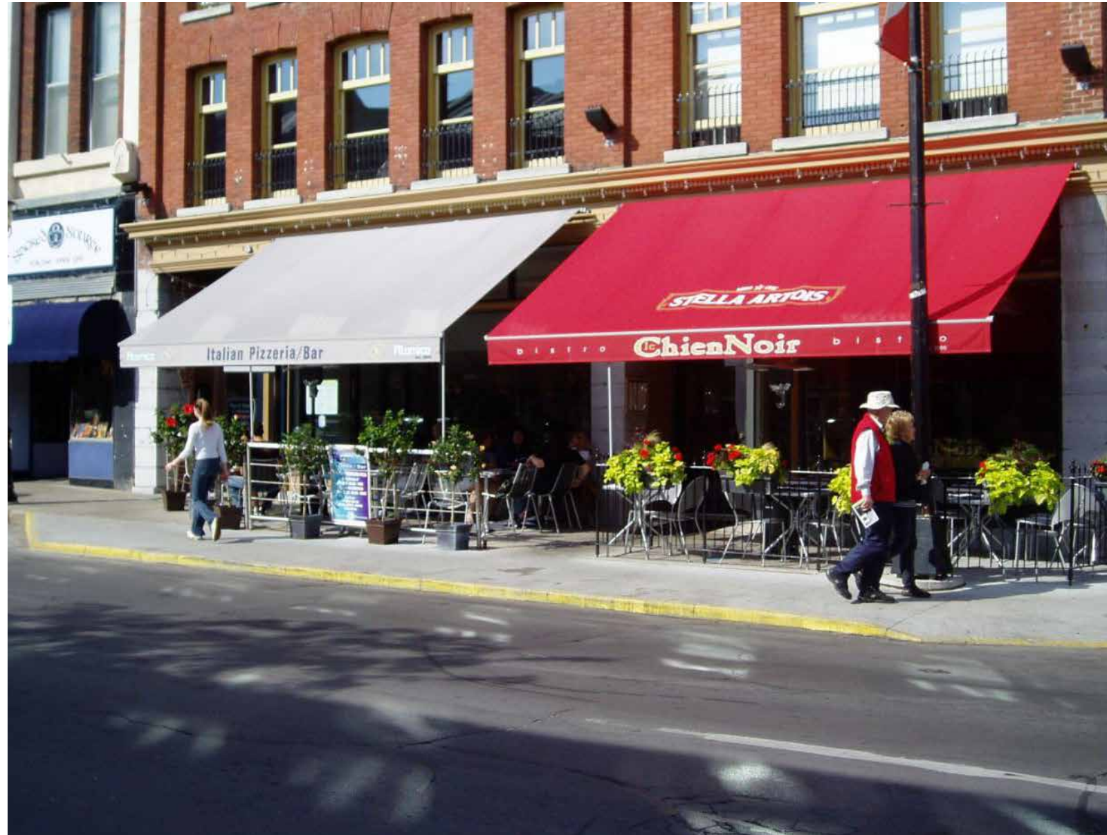
Photo of Retractable Awning at 69 & 71 Brock St, Kingston ON
