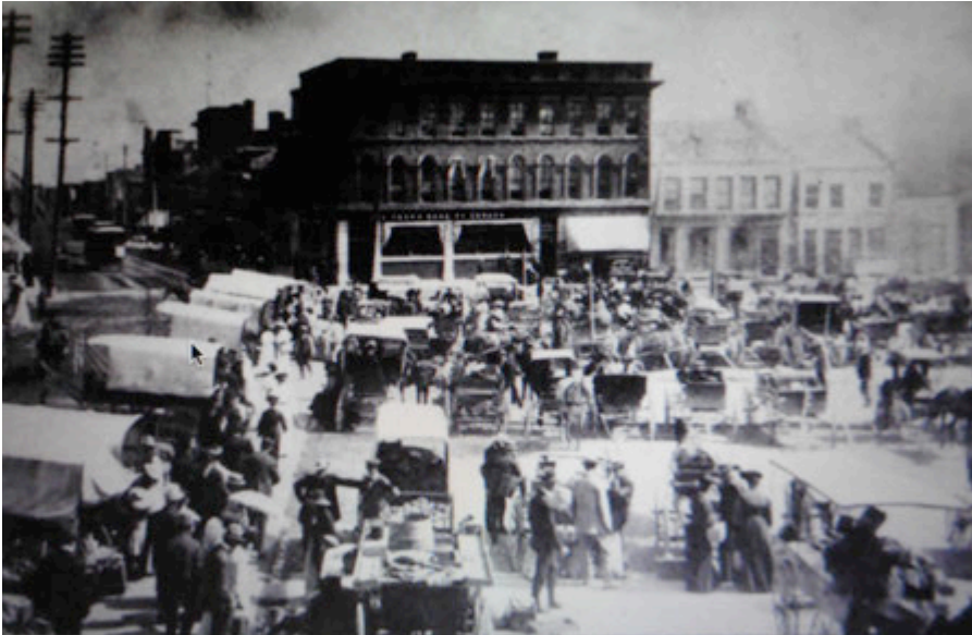
Fig. 5: 39, 35, 33 Brock Street, c.1907. Note all windows intact at 35 Brock St. (QA)
