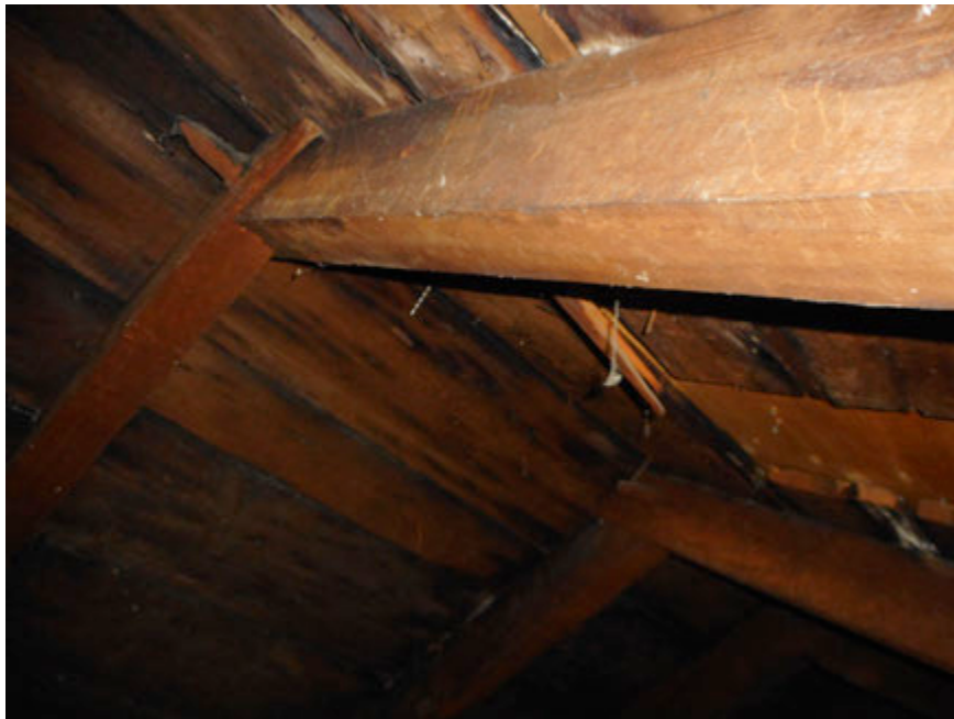
Fig.8: Rafter couples pegged at peak
