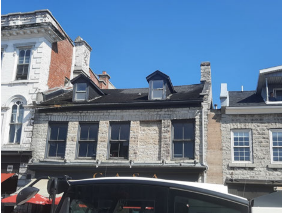
Existing Infill Wall Between 35 and 33 Brock Street
