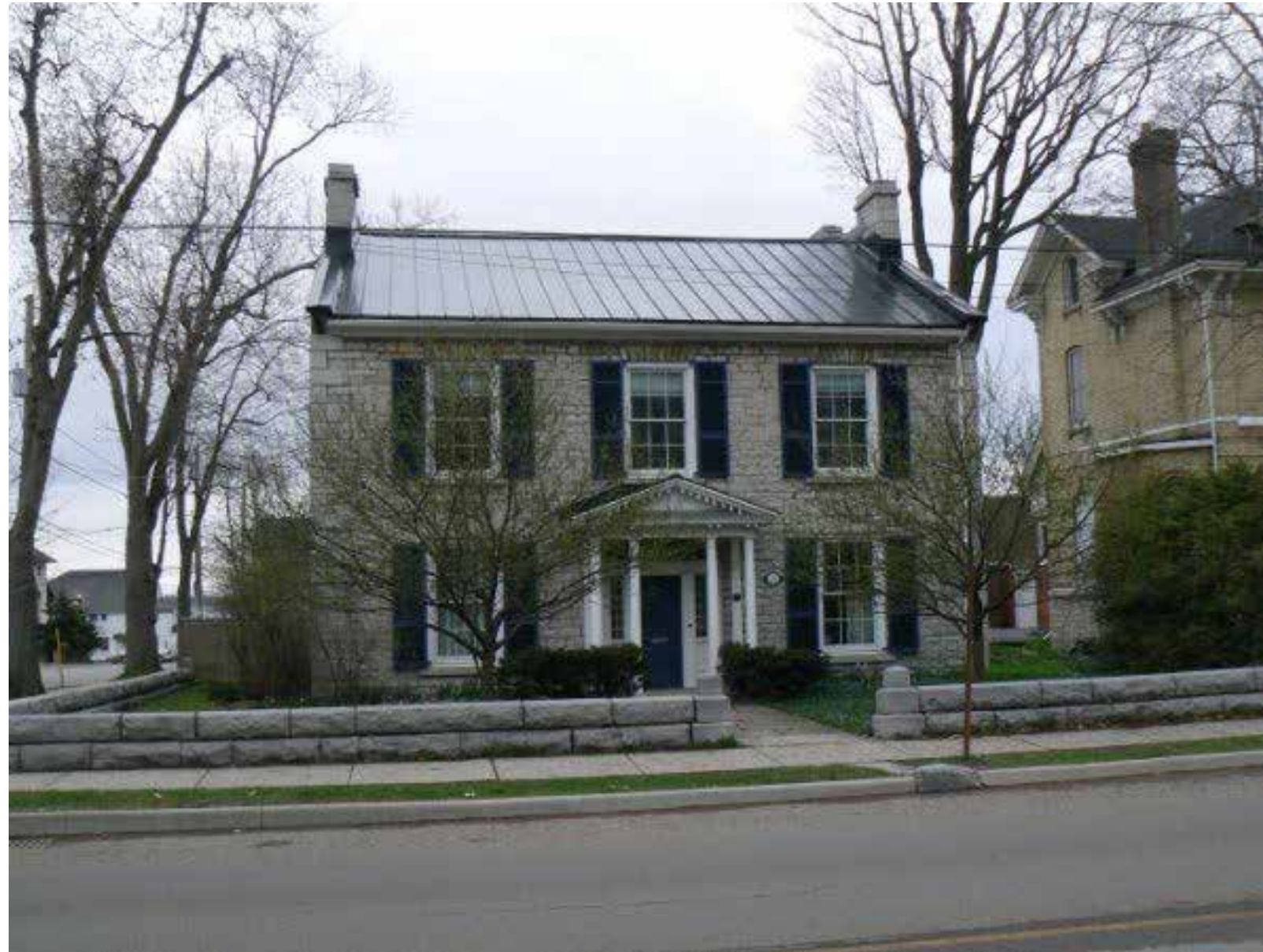
Photo of Standing Seam Metal Roof at 53 King St East, Kingston ON
