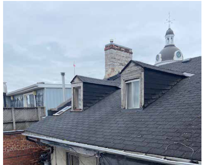
Figure 3. Shows rear portion of parapet that will be covered by addition.
