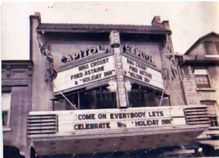
Image 6: Circa 1942 view of the upper portions of the Capitol Theatre. Note that the stepped gable parapets and pent roof are still intact, and the marquee has been replaced. Compare with Image 14.
