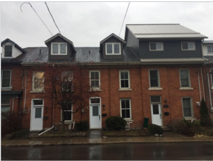
Subject properties at 29 and 31 Rideau Street
