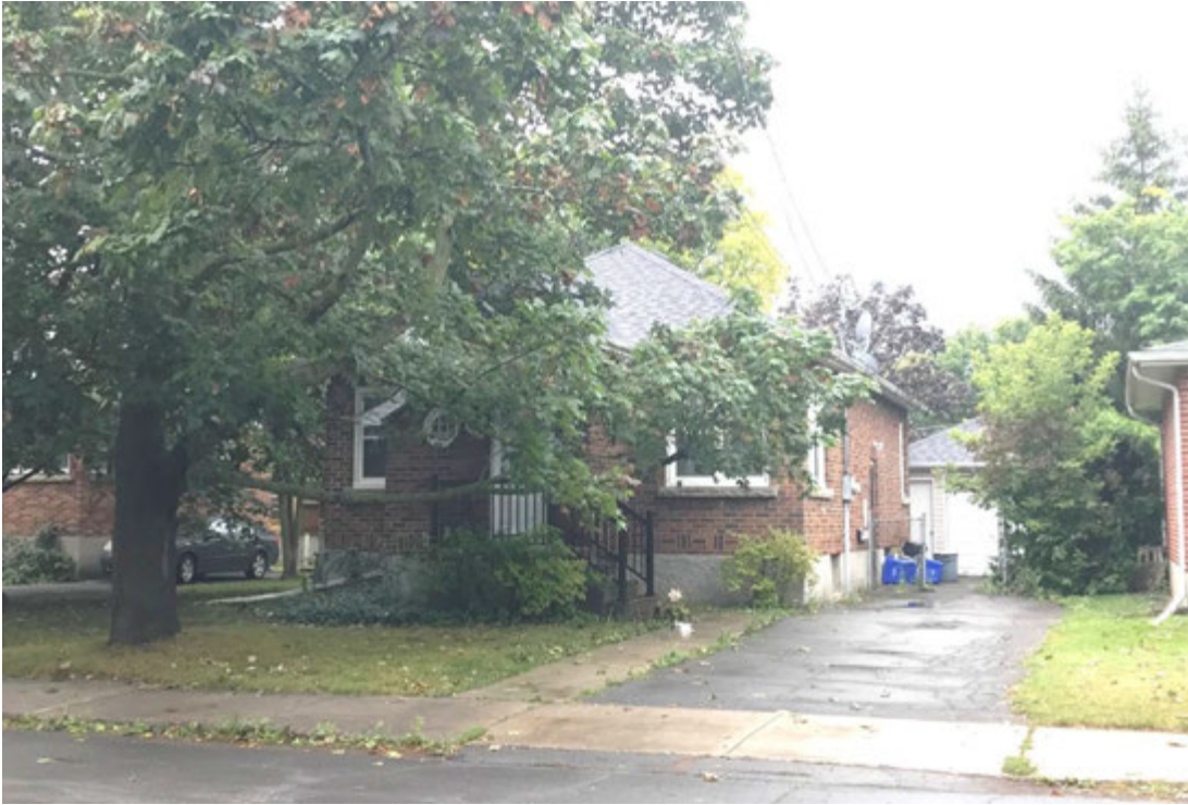
Figure 1: East facing view towards the subject property.
