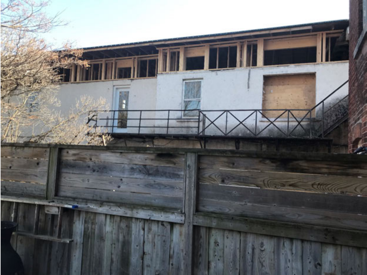
View of current fire escape from 11 Colborne street
