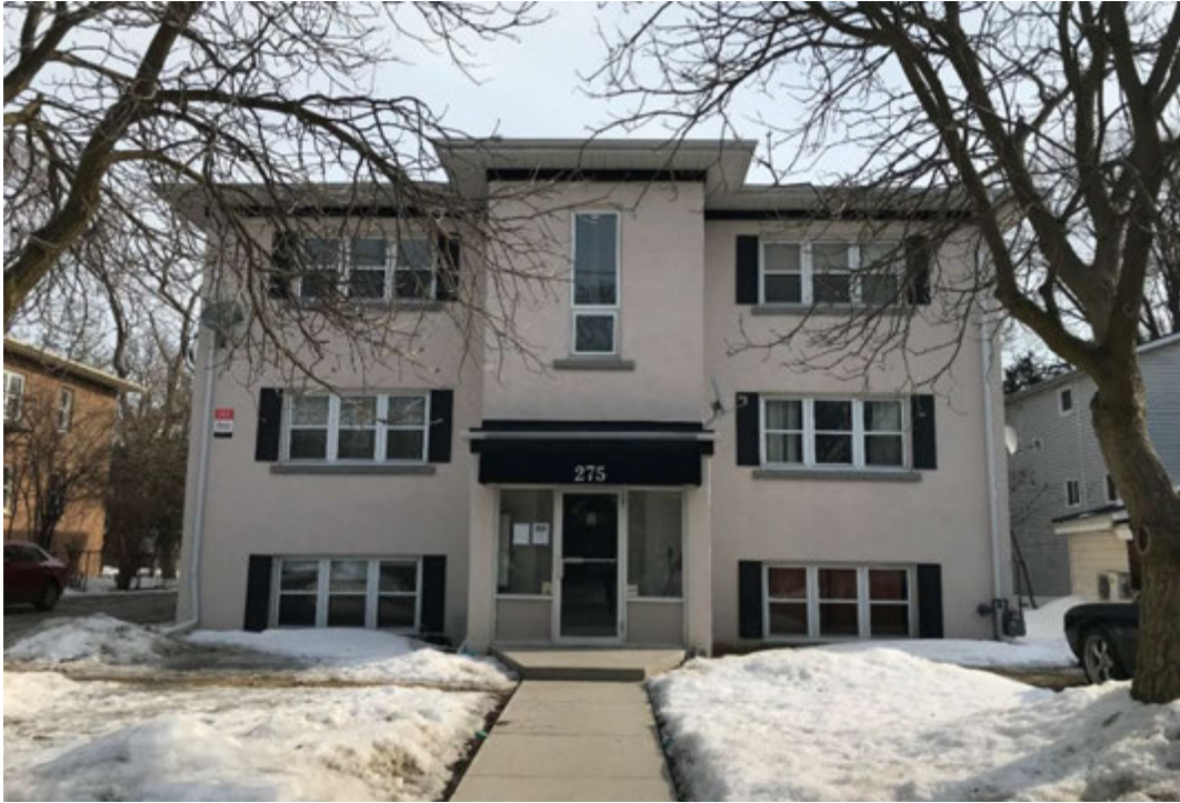
Figure 1: Existing 2.5-storey apartment building on the subject property.
