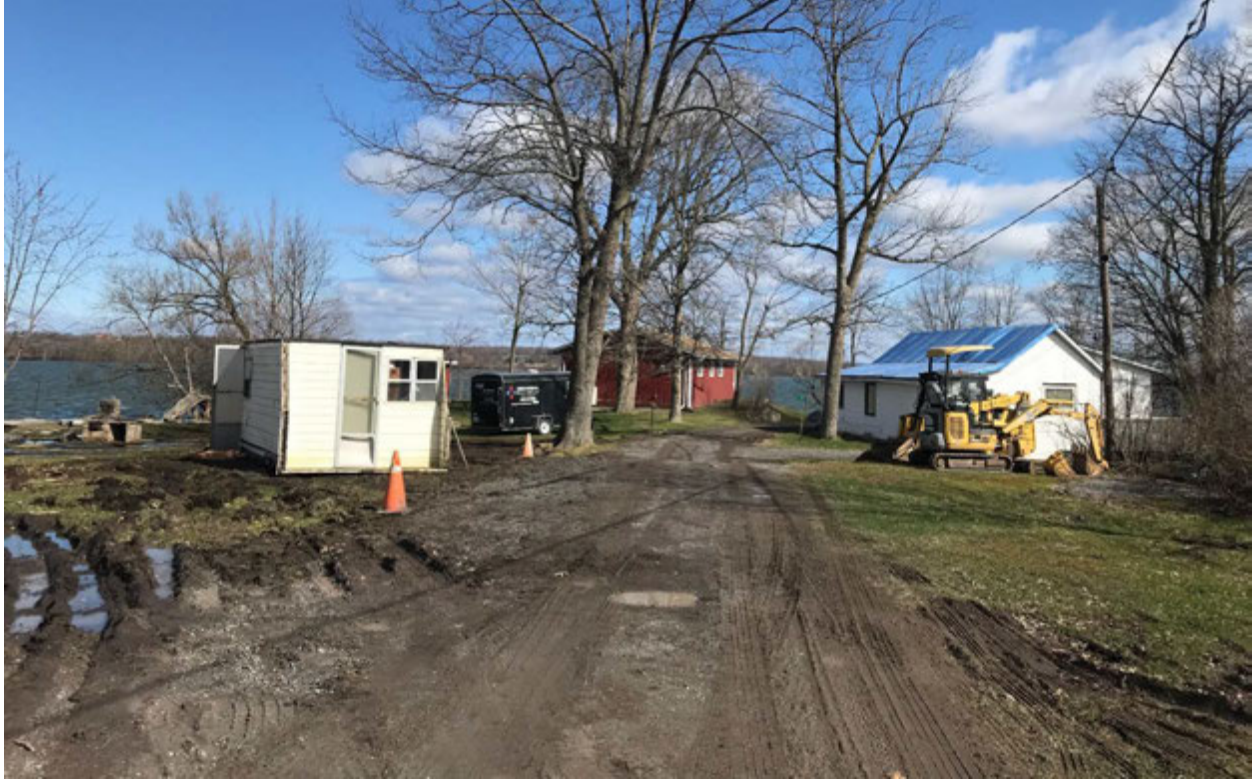
Figure 3: Site of former 8 Nina's Lane
