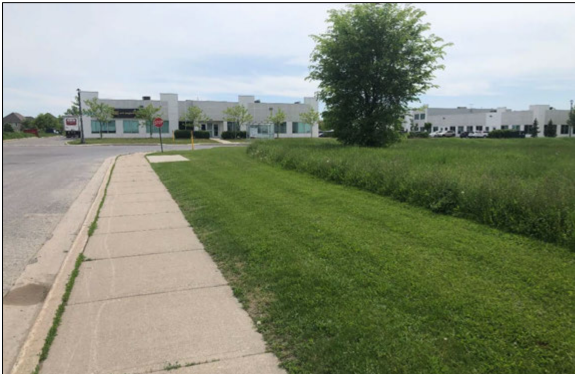
Figure 2: View of Eastern Street Frontage Looking South.
