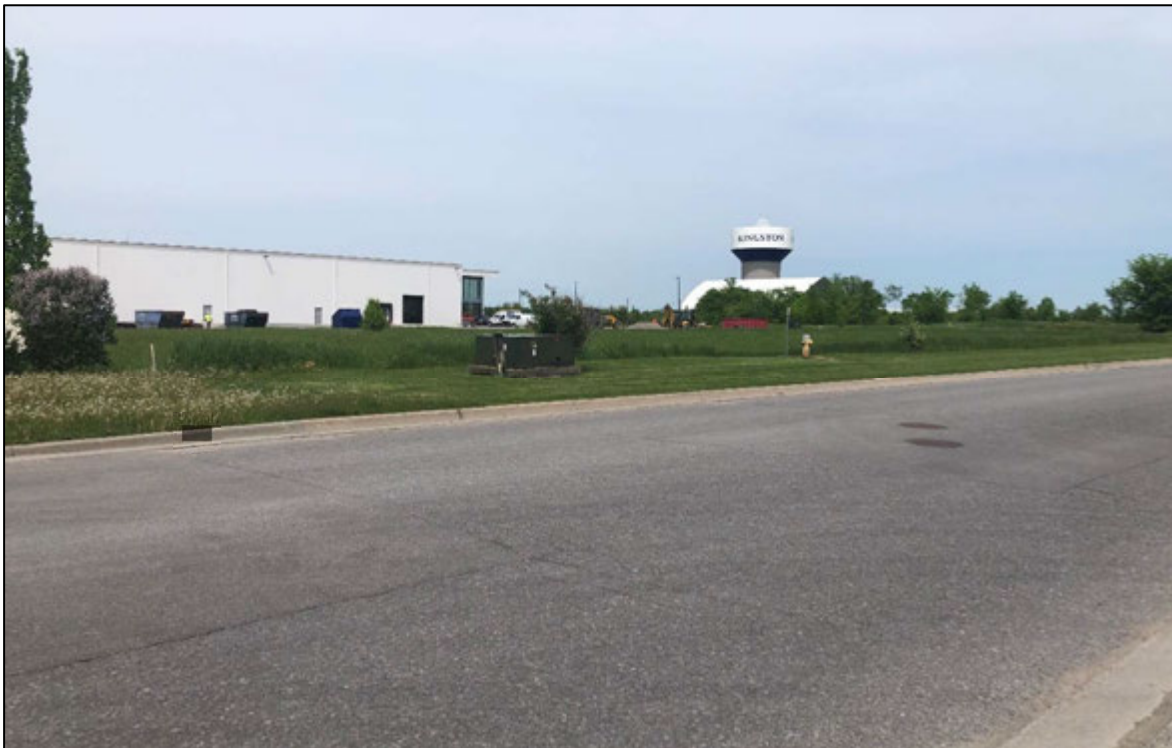
Figure 4: View of Southern Street Frontage Looking North East
