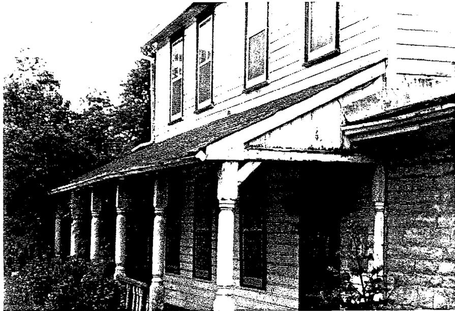
A proper roof inspection should be carried out annually. Sound flashing and operational downspouts and gutters are critical to the long term maintenance of this feature whether it is built of wood, metal or asphalt.
