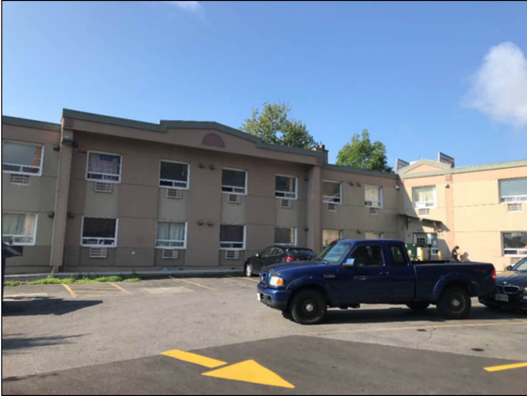
Figure 3: South facing view of the existing parking area.
