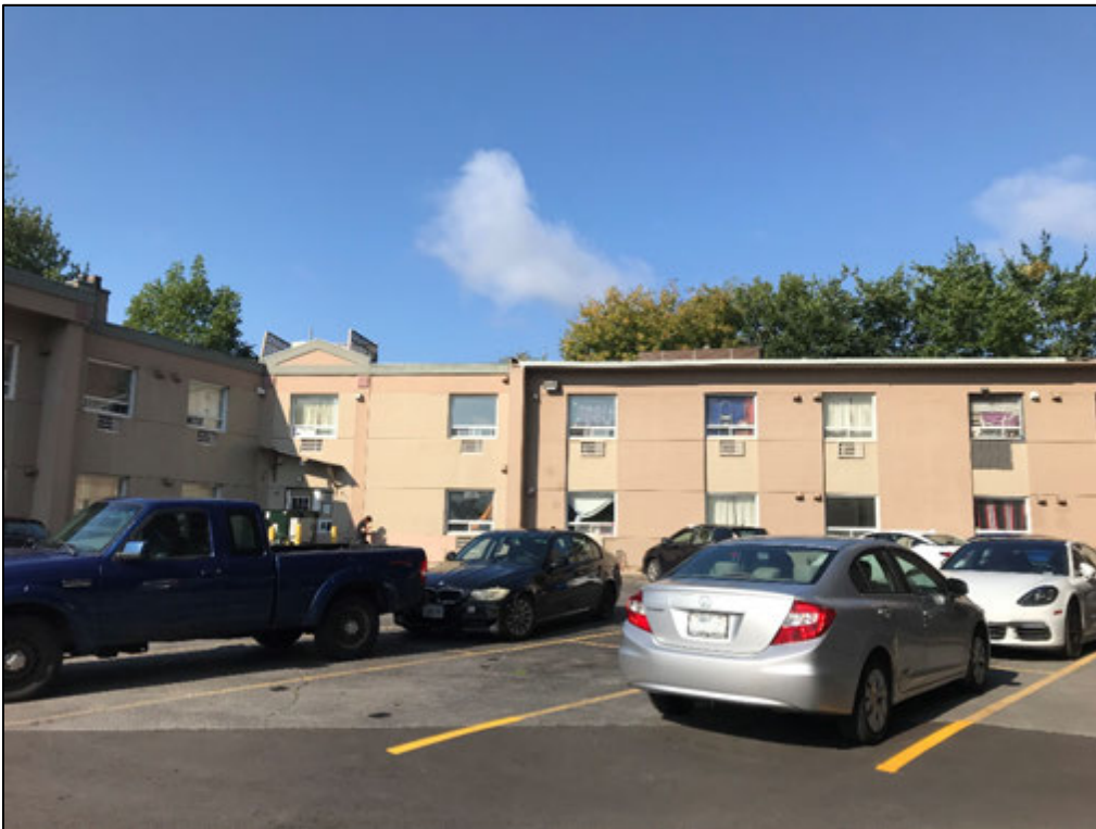
Figure 2: West facing view of the existing parking area.
