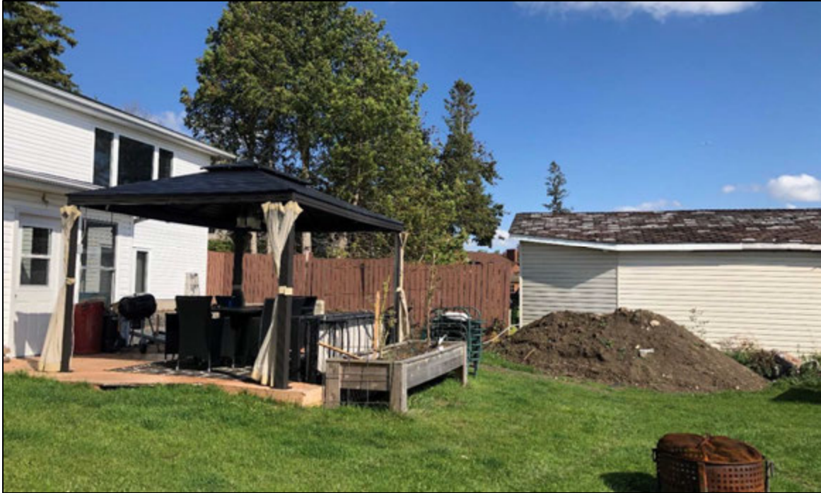
Figure 3: View of Rear of Property Facing East
