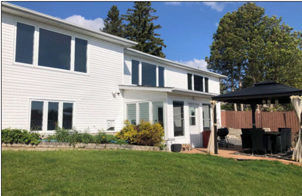
Figure 2: View of Rear of Home and Existing At-grade Sunroom.
