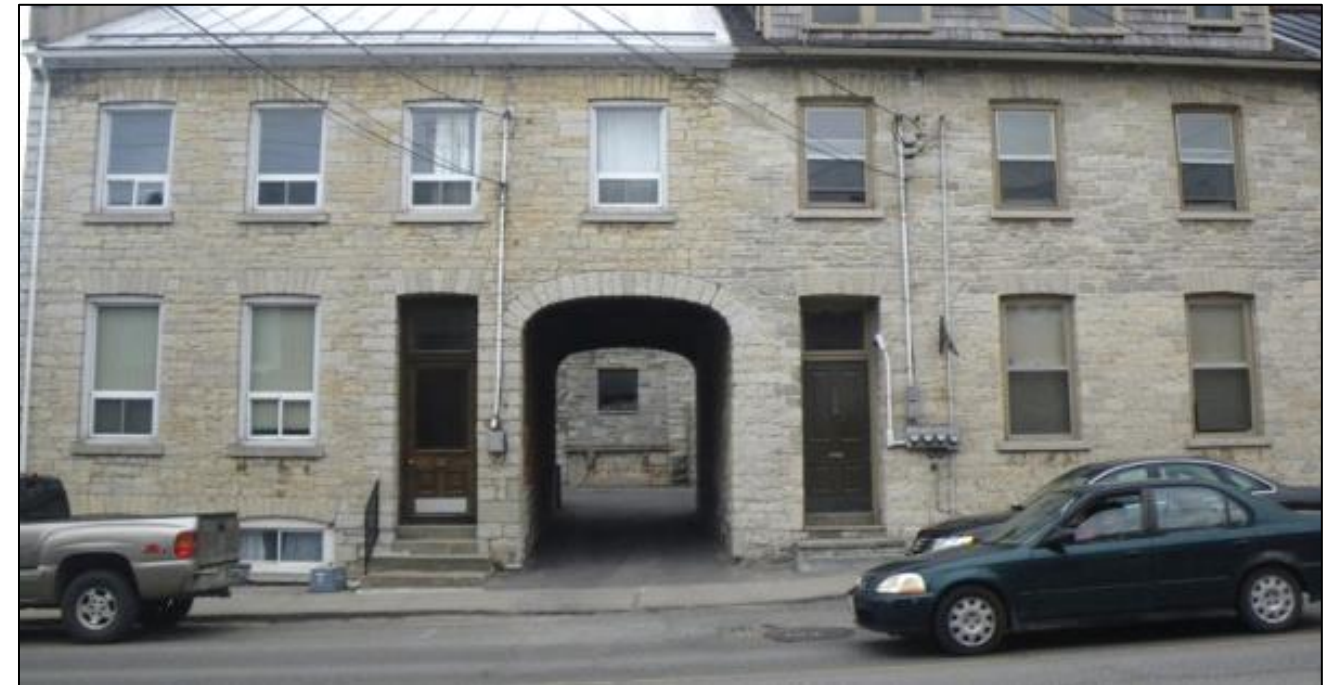
Photo 17: Existing carriage way rehabilitation, Kingston
