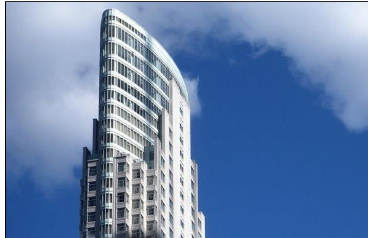
Photo 21: Refined shape of a High-Rise Building, One King West, Toronto
