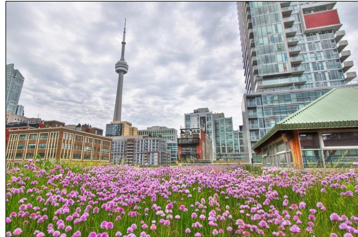
Photo 32: Mountain Equipment Co-op intensive greenroof, Toronto
