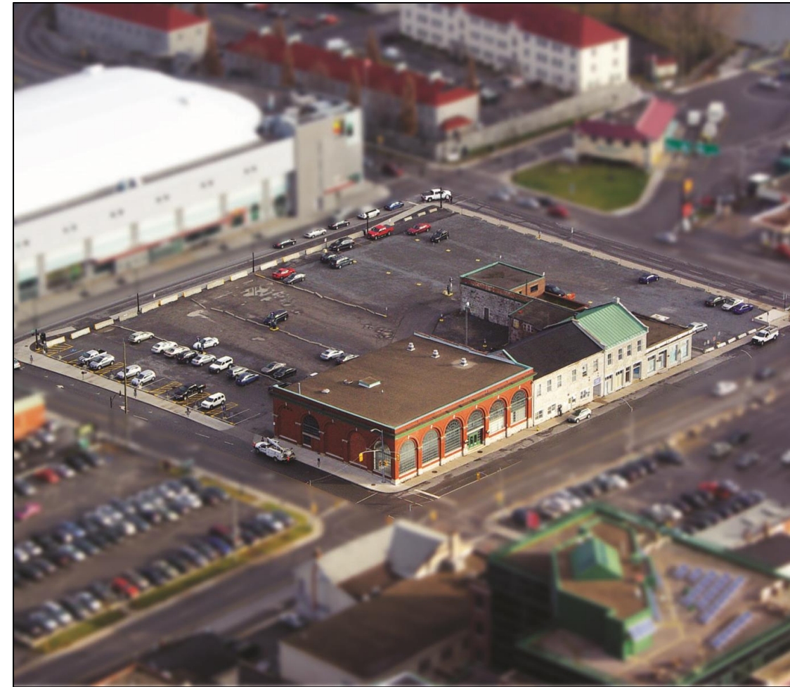
Photo 4: Existing structures on Block 4 including the Kingston Hydro substation and heritage buildings at 19, 21 and 23 Queen Street
