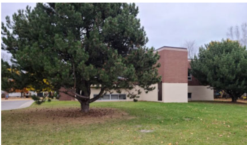
Figure 3: Eastern view of the office building. It is anticipated that removal of the two trees shown here will be required to accommodate the building expansion.
