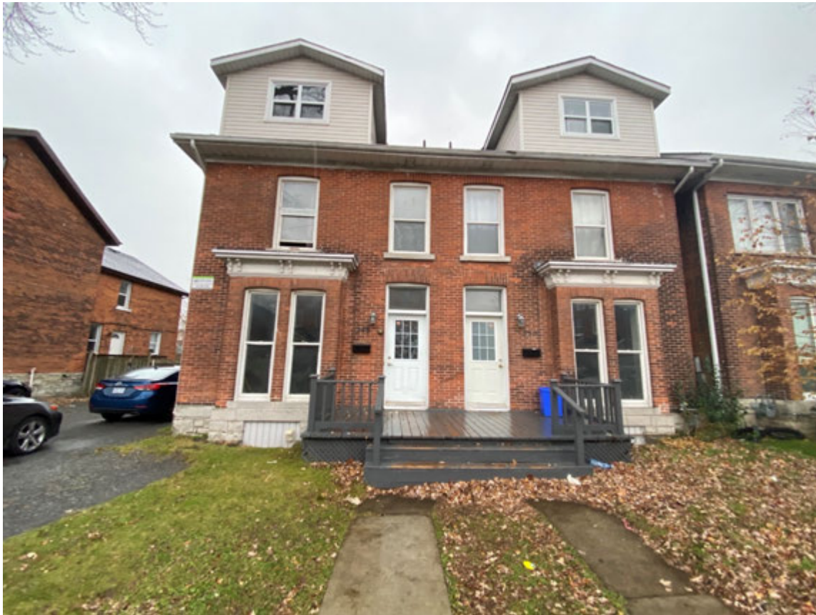
242 Alfred Street – Site photos
