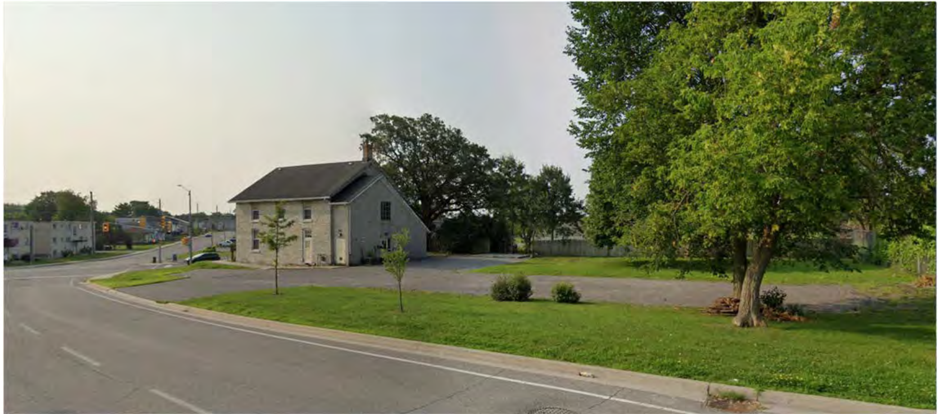
Existing heritage building with addition, and parking lot on site. View from Railway Street looking South-East
