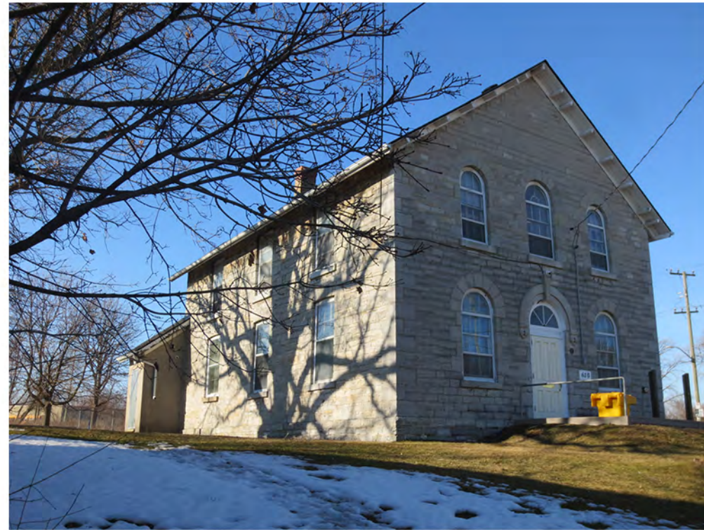
Existing heritage building exterior, view from Montreal Street
