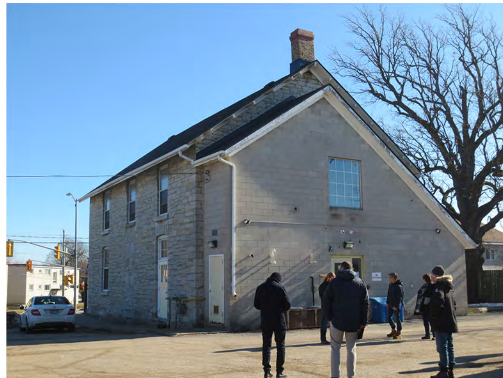
Existing addition exterior
