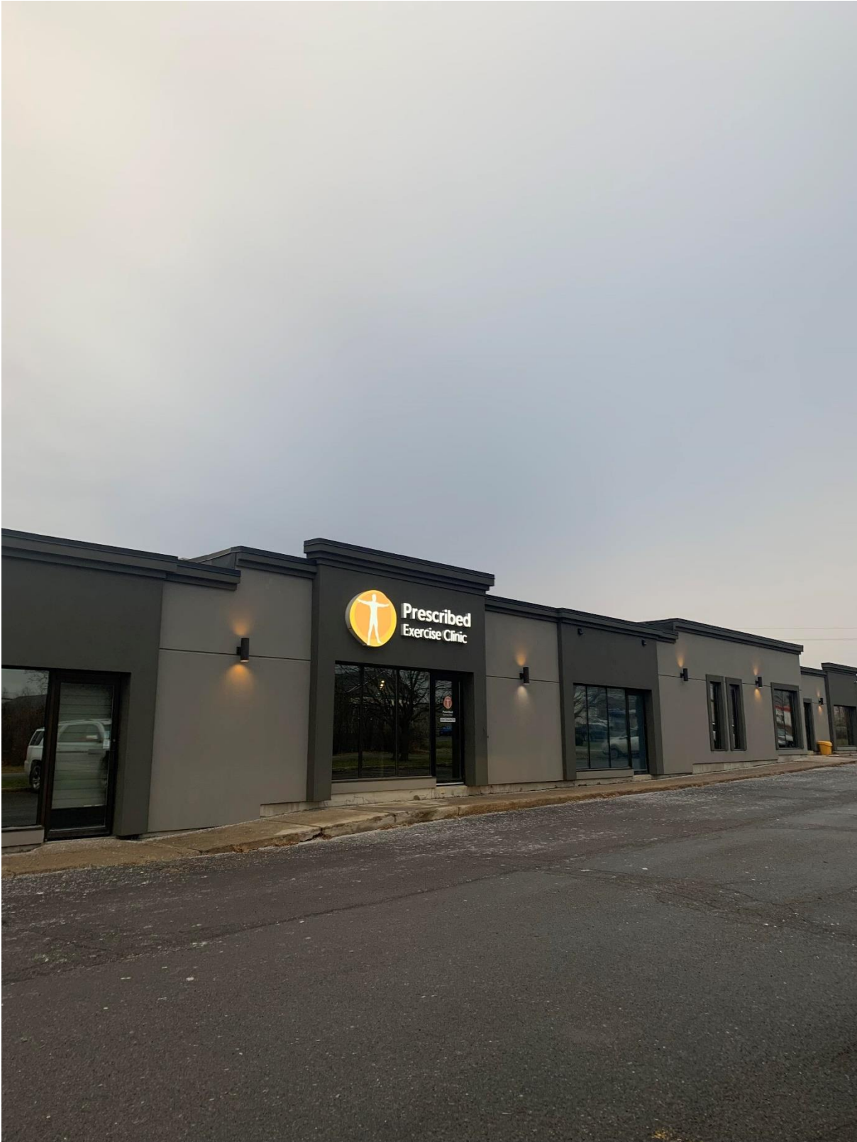
Figure 4. North facing view along Arlington Park Place, showing the existing plaza immediately across from the subject property (photo taken December 1, 2023)
