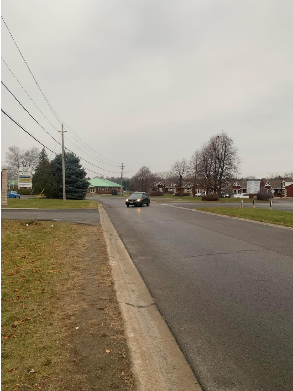
Figure 2. West facing view along Arlington Park Place frontage of the subject property (photo taken December 1, 2023).
