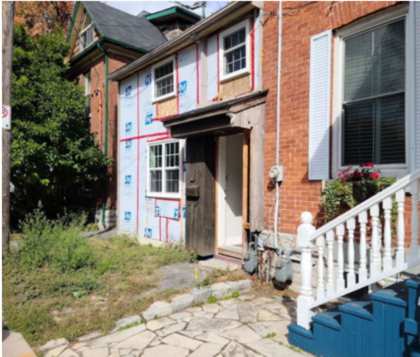
Figure 1: North-west facing view of the rowhouse at 5 York Street. A covered porch is proposed to extend outwards from the existing front wall.
