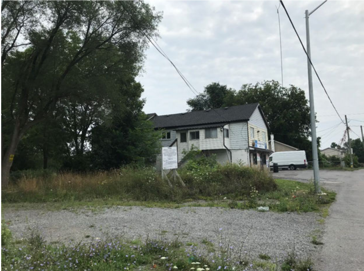
Figure 1: The upper portion of the subject site (foreground, with zone-change sign shown), viewed from along Montreal Street, looking south. A neighbouring property containing a small grocer is shown beyond.
