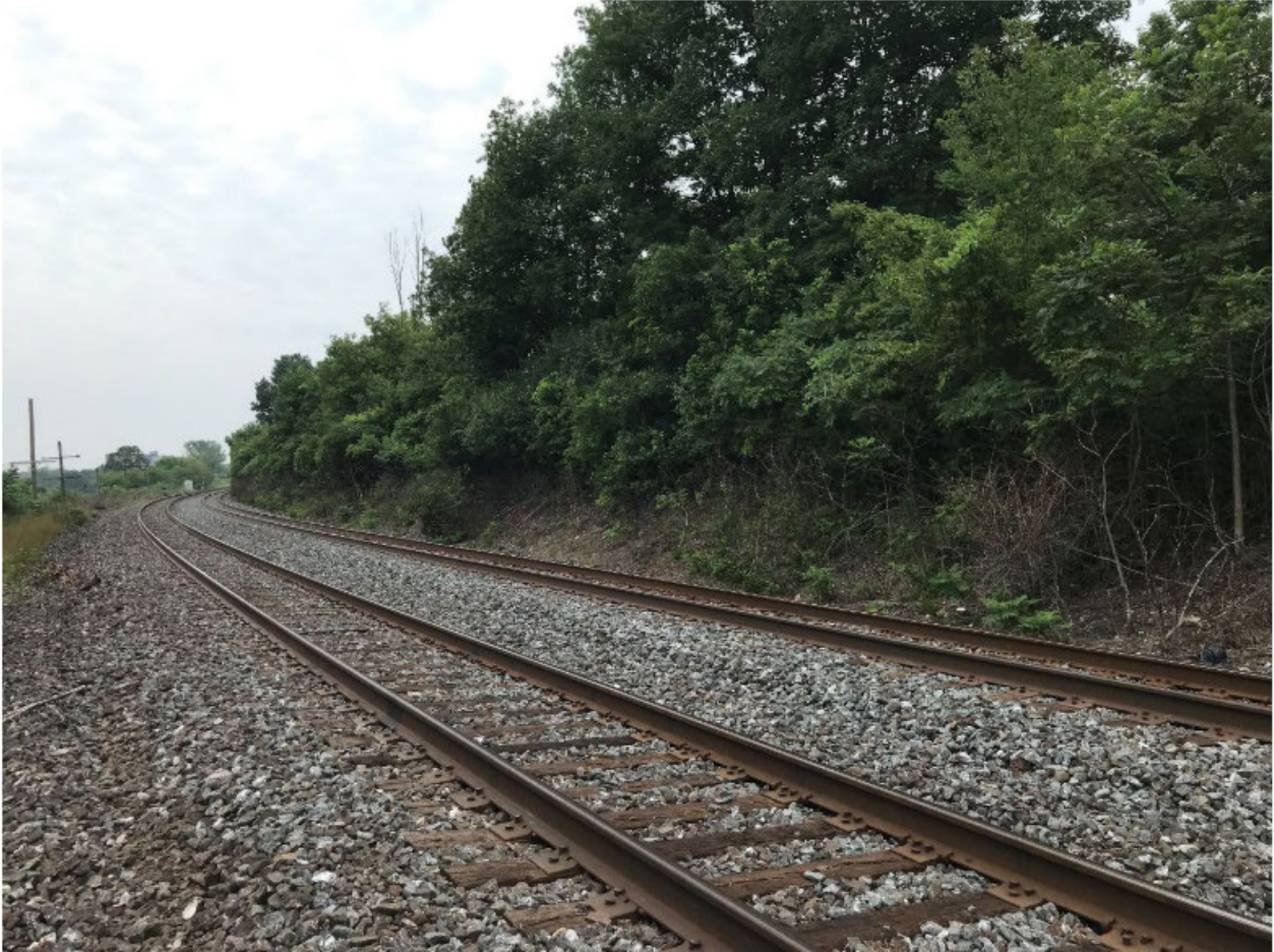
Figure 5: The CN rail line, looking south, abuts the eastern boundary of the site, pictured here to the right. The development will be set back 30 metres from the rail corridor, within which a treed berm is proposed for enhanced safety measures, along with the already significant grade change between the property and the railway.
