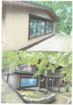
Roof top Deck with Foundation
