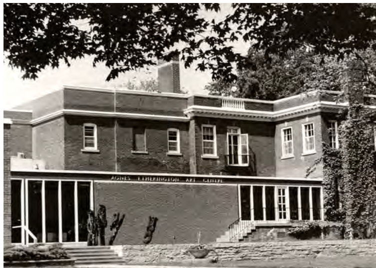
86. Archival photo of AEAC showing 1-over-1 storm windows at second floor of the Historic House
