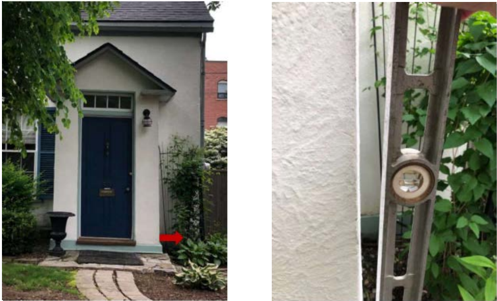
These photographs show the bottom of the side wall three inches out of plumb.
