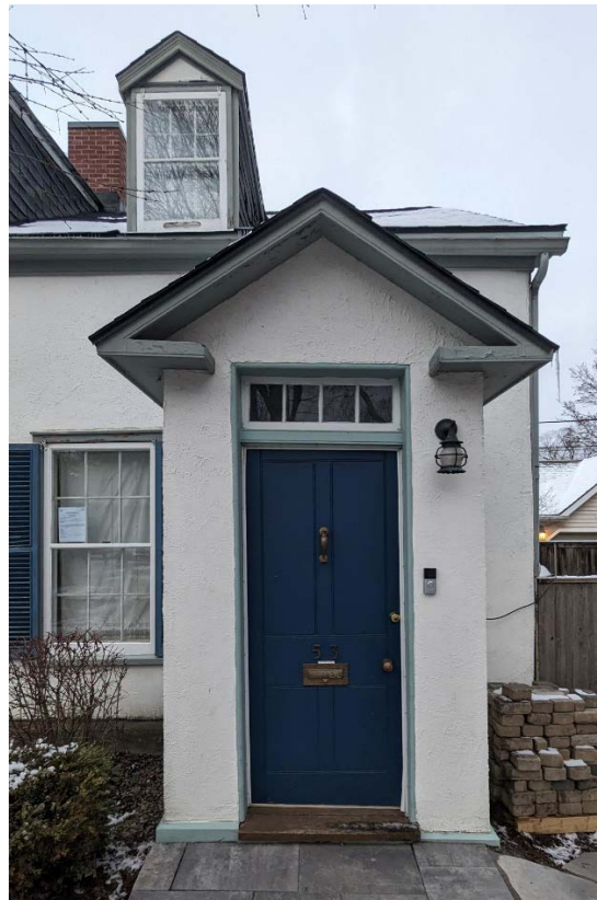
Below: Entryway vestibule head on.
