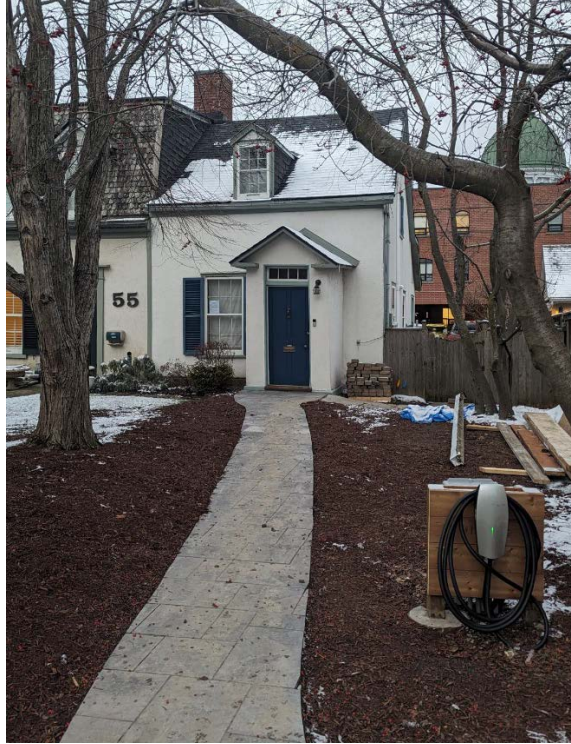
Above: Entryway vestibule from driveway.
