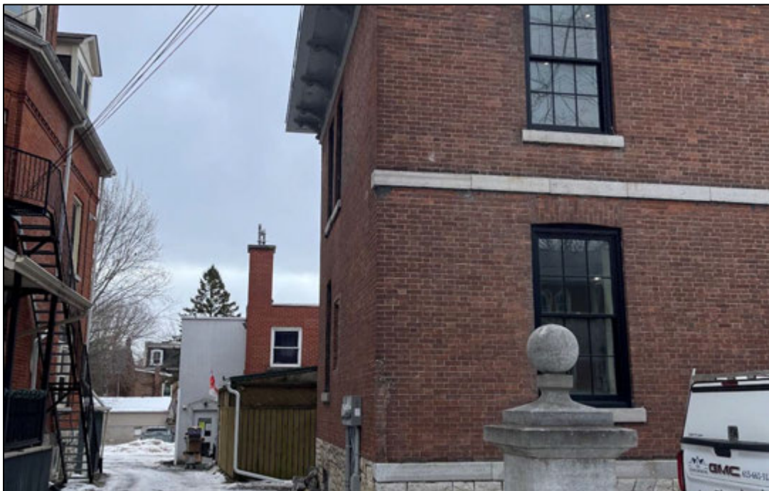
Figure 2: View of rear lane from Bagot Street
