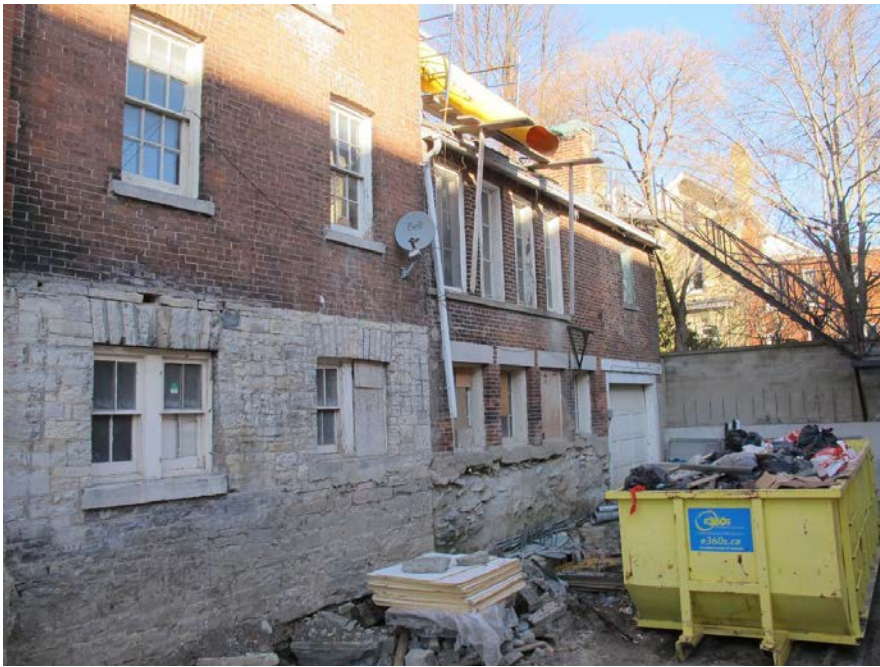
Subgrade conditions on hotel and courtyard
