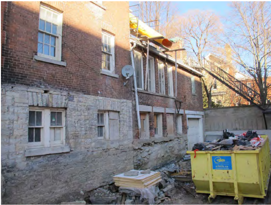
Subgrade conditions on hotel and courtyard
