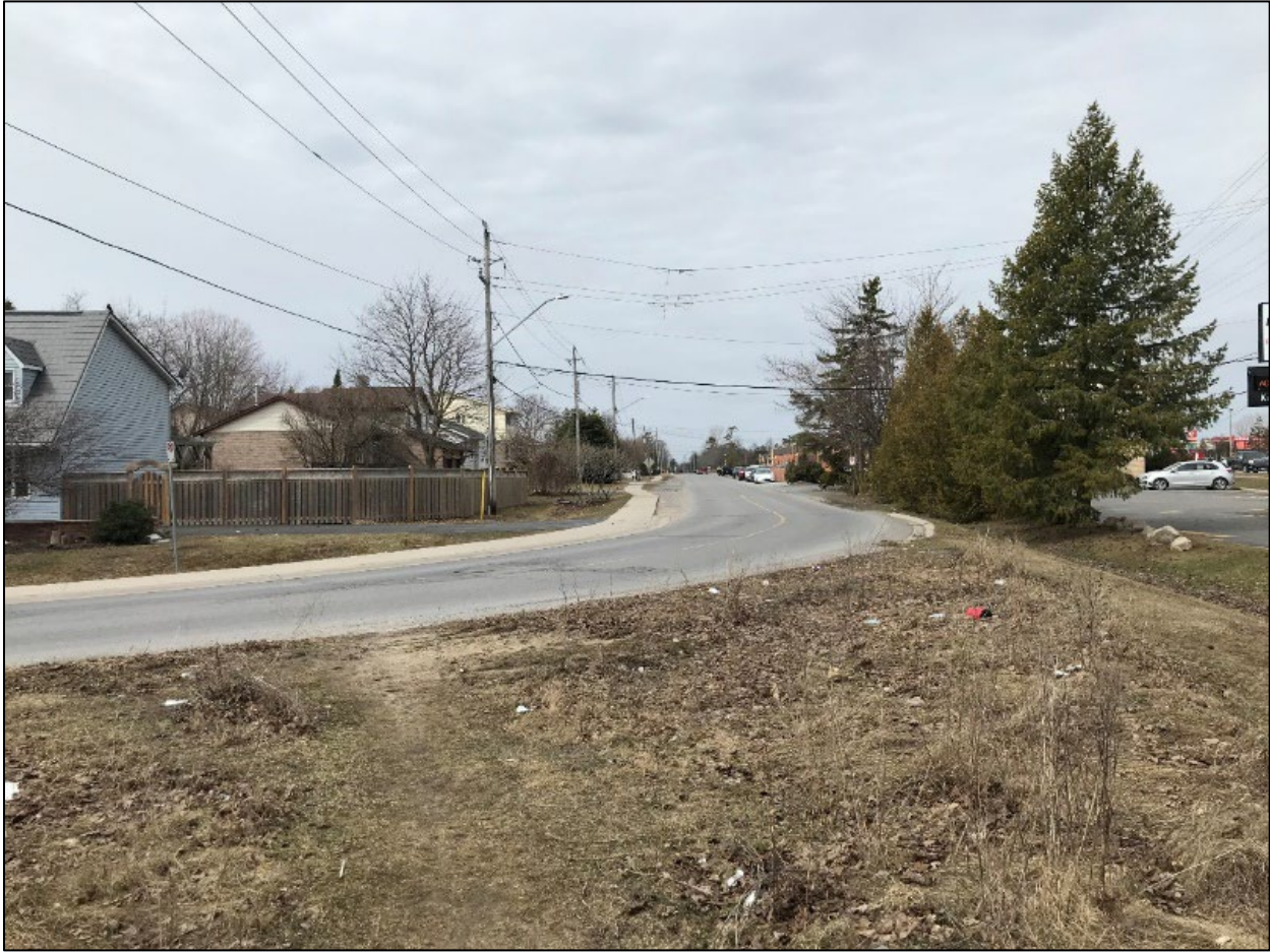
Figure 9: Woodbine Road, viewed looking west. The subject site is to right (north), behind the trees standing along its southern property line.
