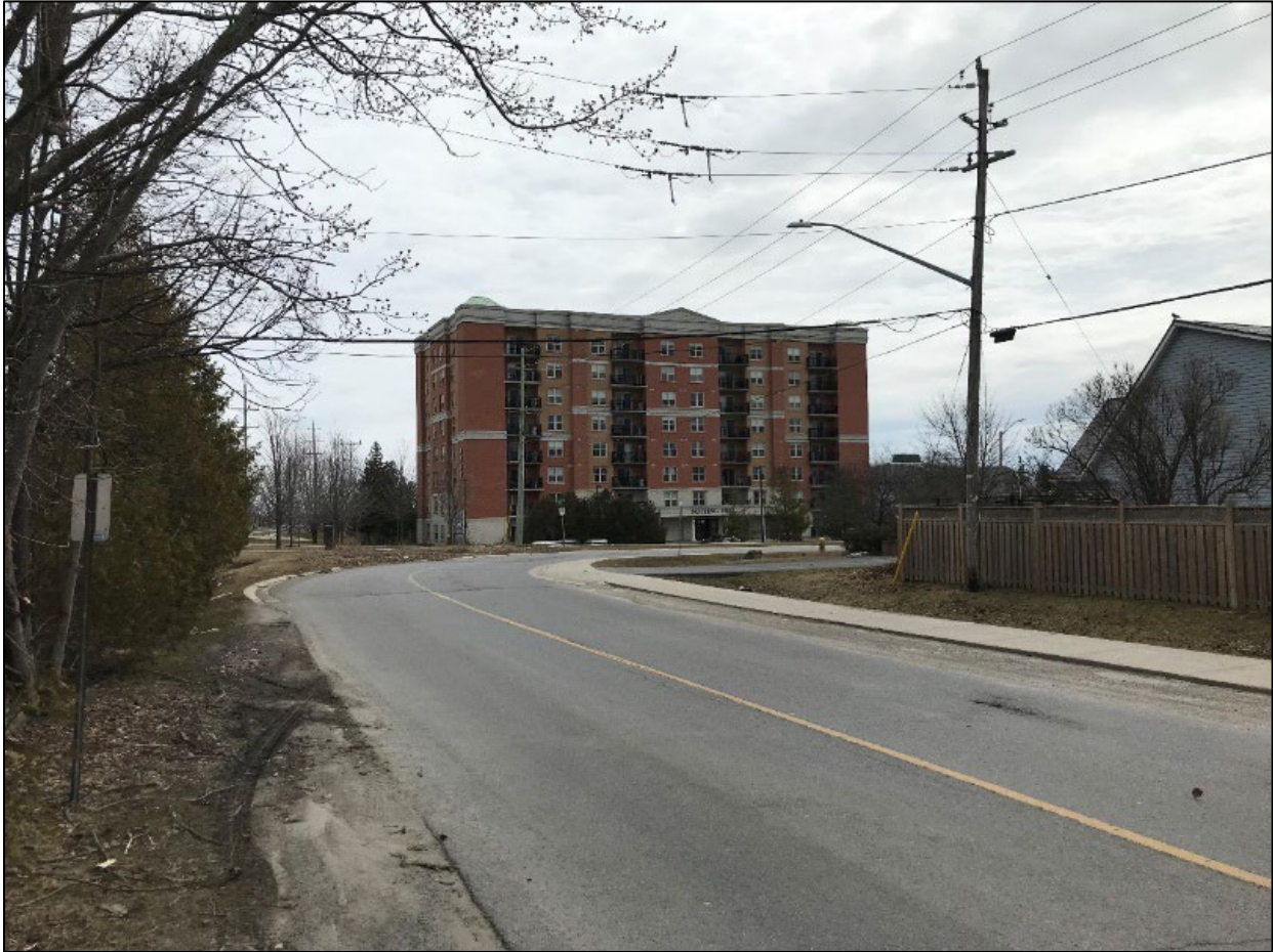
Figure 10: The eight-storey apartment building situated to the east of the subject property (located beyond the row of trees to the left of the image). The apartment building is accessed from both Princess Street and Nottinghill Avenue, which transitions into Woodbine Road (pictured in the foreground).
