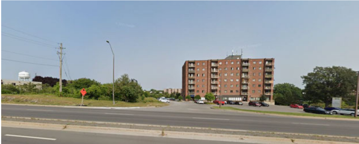
From Gardiners Road looking east, with existing apartment building and parking area to the right and vacant portion of the lands to the left.
