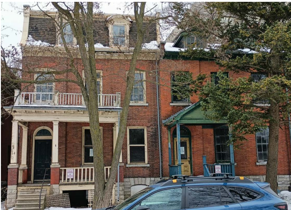
Doran & Robinson Houses – 64-66 Barrie St
