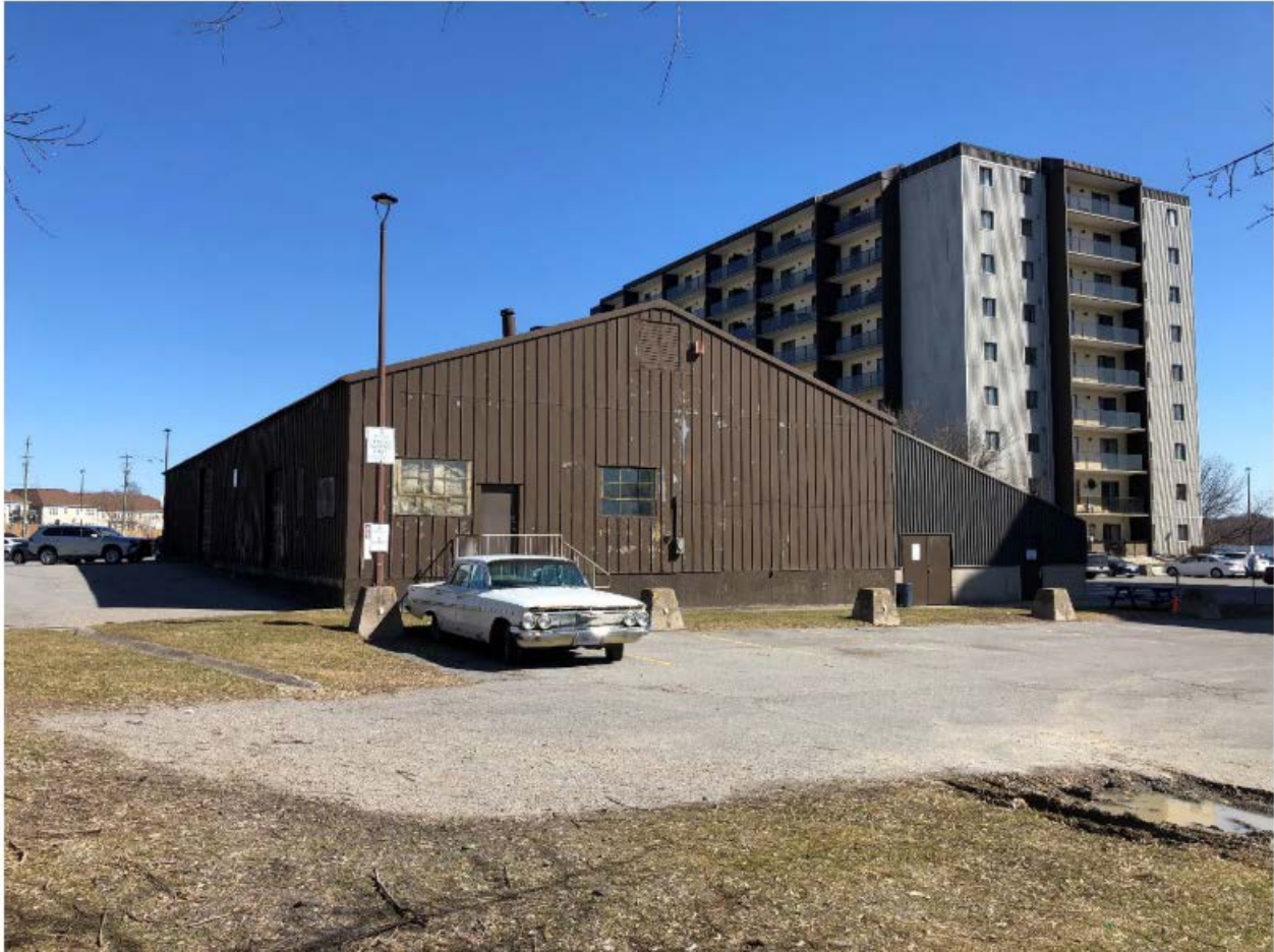
Figure 5: Significant parking lot improvements are planned for the area currently occupied by the large storage building, which would be removed. These improvements would not only provide additional resident parking, but would enhance aesthetics and enable better connectivity throughout this area.
