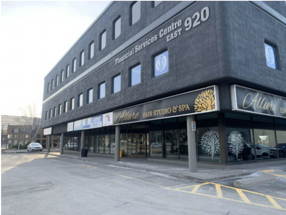
Figure 6. The existing building addressed as 920 Princess Street on the subject property, which includes a variety of commercial opportunities (photo taken March 22, 2024).
