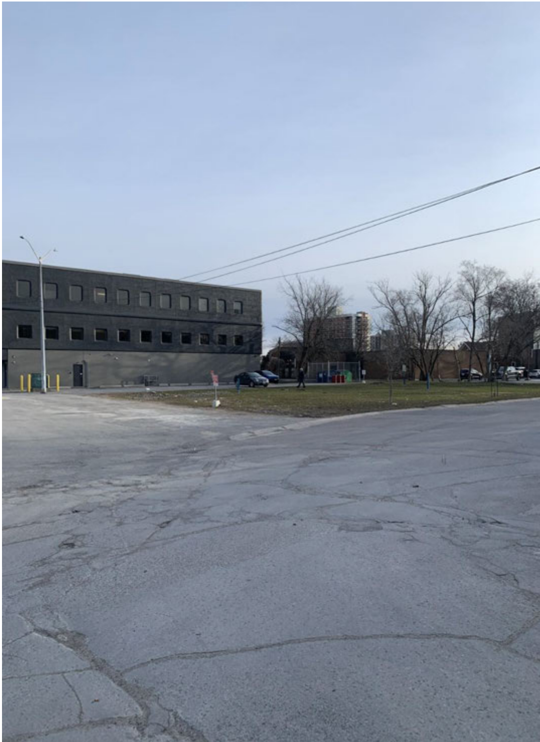
Figure 1. North facing view along Franklin frontage of the undeveloped portion of the subject property (photo taken March 22, 2024).
