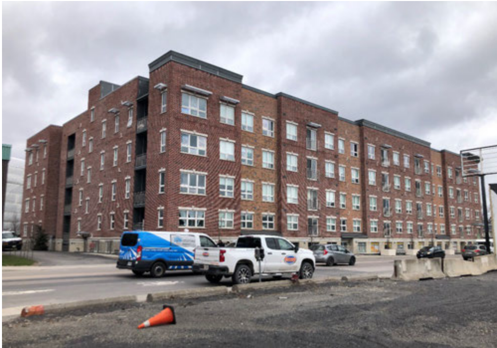
Figure 1: Princess Street (south) and side (west) elevations.
