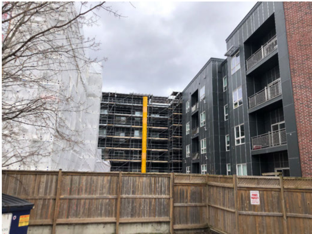
Figure 4: Rear interior courtyard.
