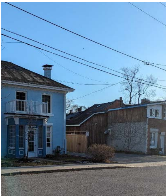
Above: Looking towards the rear of 160 Bagot Street from Lily Lane on Earl Street.
