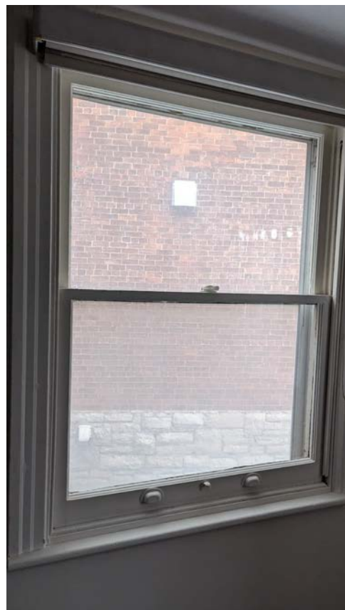
WINDOW 4 MAIN FL EAST
