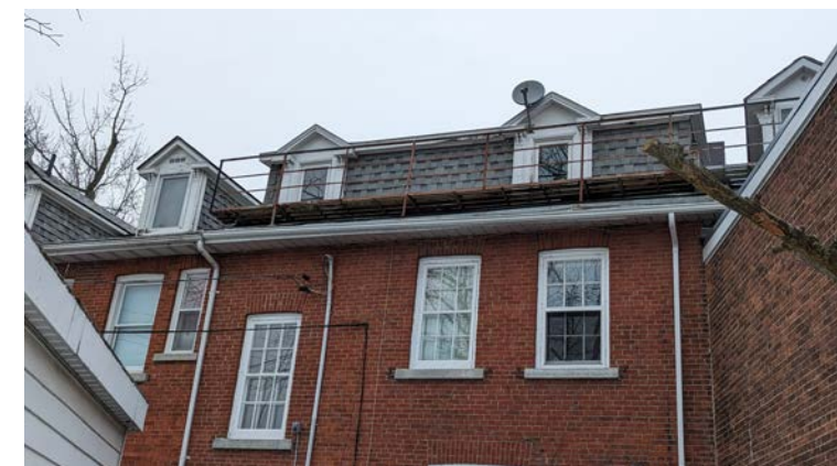
SOUTH SHED DORMER at 160 EARL
