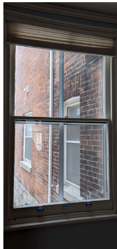
WINDOW 2 MAIN FL SOUTH
