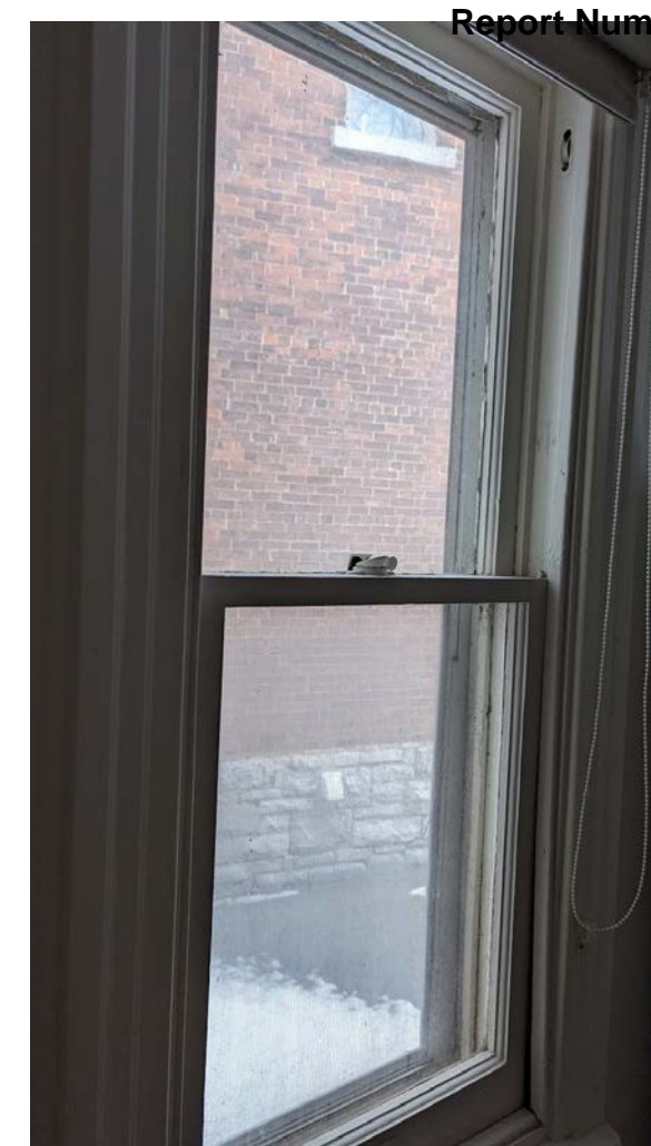
WINDOW 3 MAIN FL EAST
