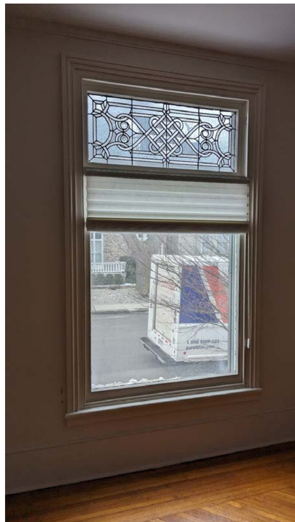
WINDOW 1 MAIN FL NORTH
