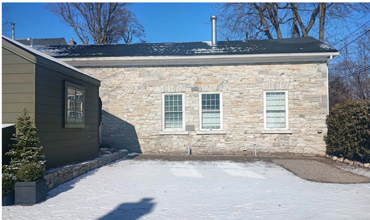
Looking north towards the east elevation of the shed and the south elevation of the adjacent stone outbuilding.
