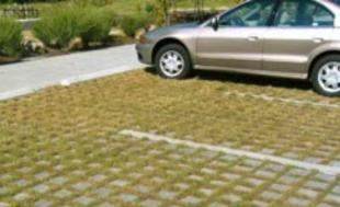
Figure 6-3: (Left) Landscaped islands delineate the parking areas, and trees provide shade and reduce heat island effects. (Right) Permeable surface treatments, including permeable pavers or asphalt, should be considered to promote on-site water retention, thus reducing dependency on the City's storm sewer and combined sewer system.
