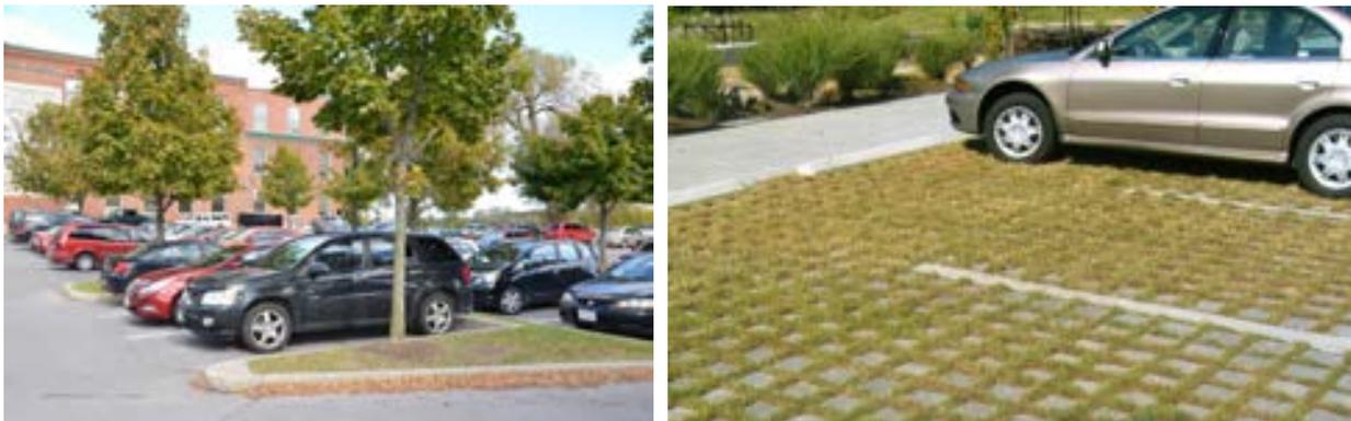
**Figure 6-3:** (Left) Landscaped islands delineate the parking areas, and trees provide shade and reduce heat island effects. (Right) Permeable surface treatments, including permeable pavers or asphalt, should be considered to promote on-site water retention, thus reducing dependency on the City's storm sewer and combined sewer system.
