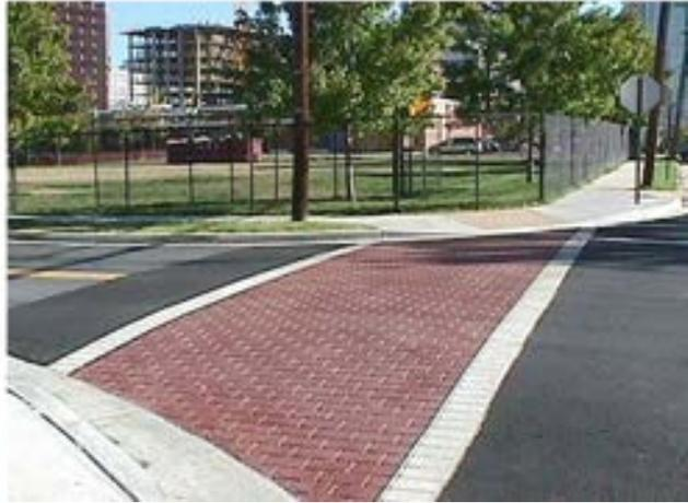
**Figure 5-16:** Crosswalks are clearly-defined, properly graded and connected to the sidewalk network. Defined crosswalks remind users of pedestrian priority.
