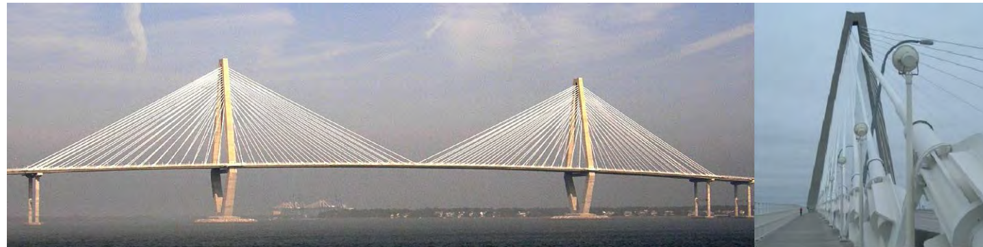
New Cooper River Bridge, SC
