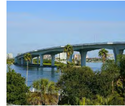
Clearwater Bridge, FL
