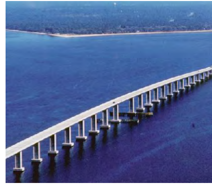
Mid-Bay Bridge, FL
