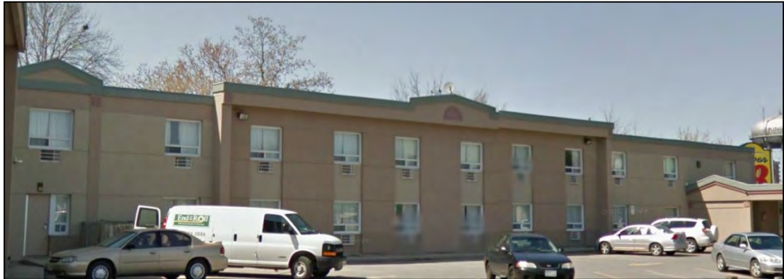
Figure 9: East elevation of original (north) wing of existing structure (Source: Google, 2013).
