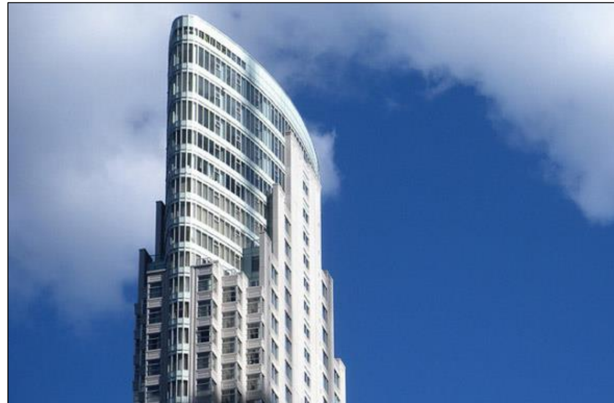
Photo 21: Refined shape of a High-Rise Building, One King West, Toronto
