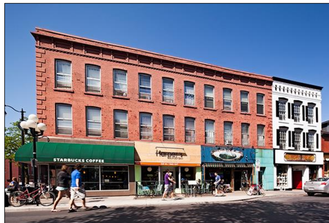
Photo 8: Active retail frontages on Princess Street in Kingston with functional building entries at 10-20 metres or less
