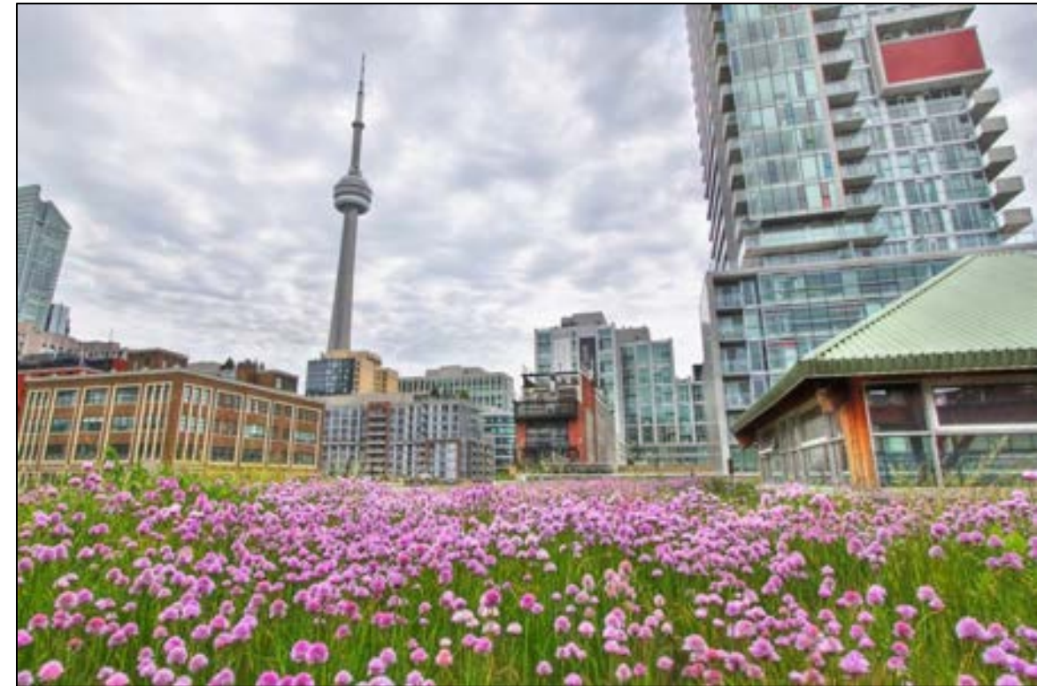
Photo 32: Mountain Equipment Co-op intensive greenroof, Toronto
