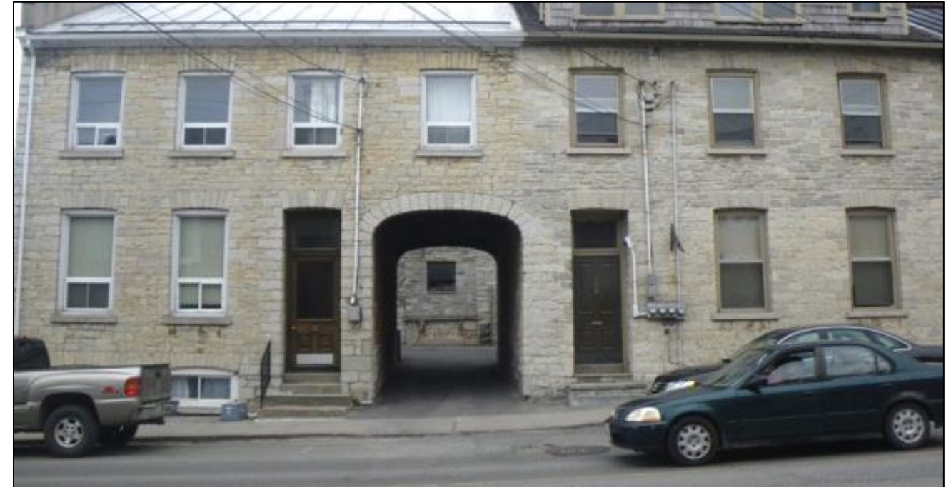
Photo 17: Existing carriage way rehabilitation, Kingston
