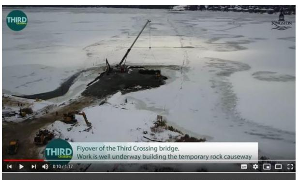
An aerial video of construction work on the east and west shores and in-water work building the temporary rock causeway and the first of five wildlife passages.
