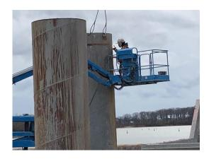
Image on the left below: The image on left below shows the completed shafts with all the reinforcing steel and concrete that has been placed inside the steel casings. The two completed shafts are now ready to receive the pier cap.
